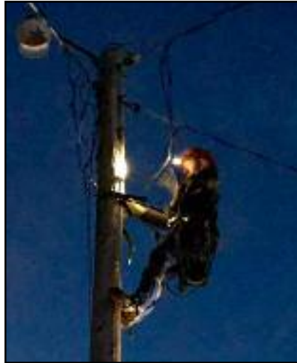
Ben Hager working after hours to restore power after a storm
