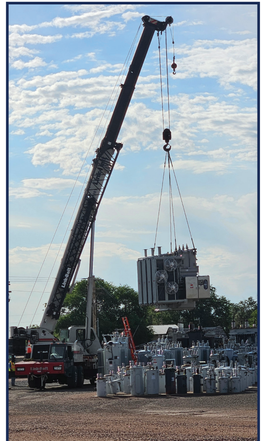
A 10 mva transformer, weighing 66,000 lbs, is being lifted onto a truck to be taken for repairs
